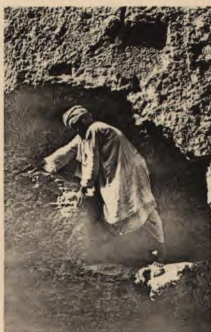
7. THE WORKMEN'S STAIRS.
