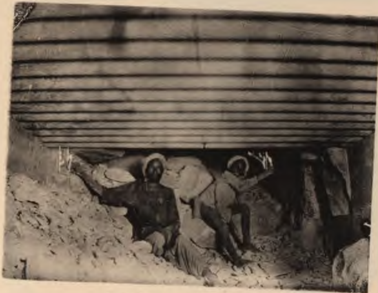
1. POLE ROOF, CHAMBER C.
